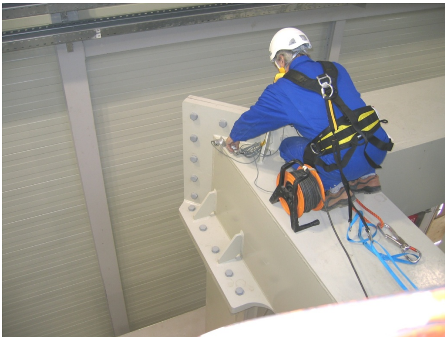
Figure 5: Mounting of sensors on top of steel frame
